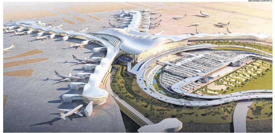
Building the future: construction consultancy Turner & Townsend designed Abu Dhabi international airport and is advising on the creation of Qatar's new coastal city, Lusail
